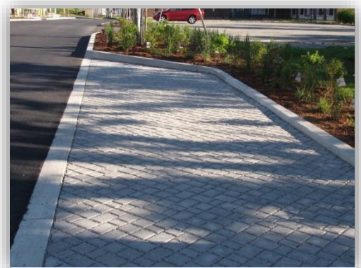
Example of permeable pavers for a parking lane in Yarmouth
