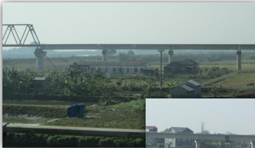
Example of road raised above the floodplain and dyke system – (Red River, Vietnam)
