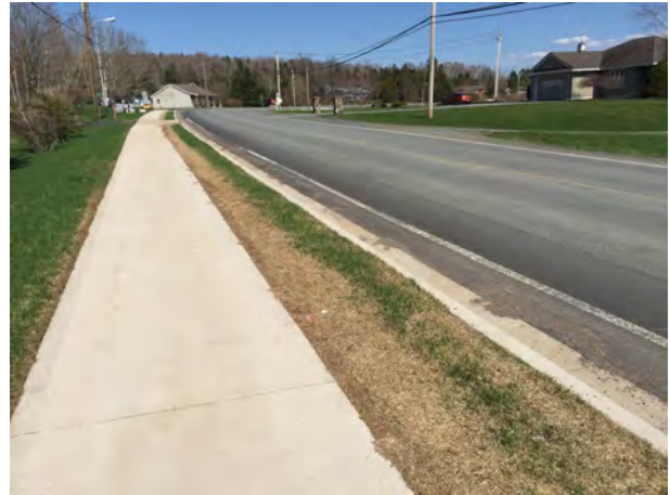
Sidewalk Project, Highway 289 (Brookfield)
