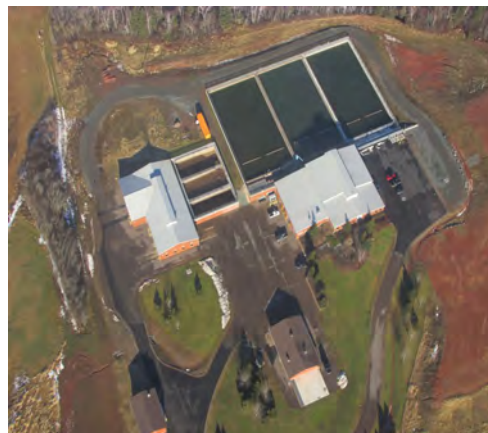
Central Colchester Wastewater Treatment Facility
