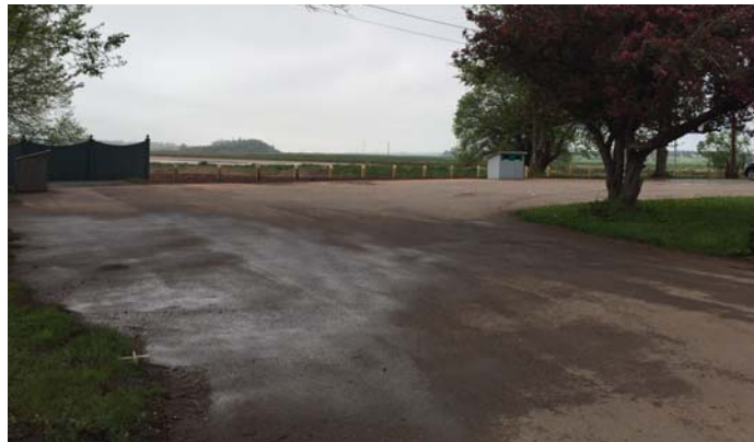
Grounds improvements happening at the former Palliser Property.
