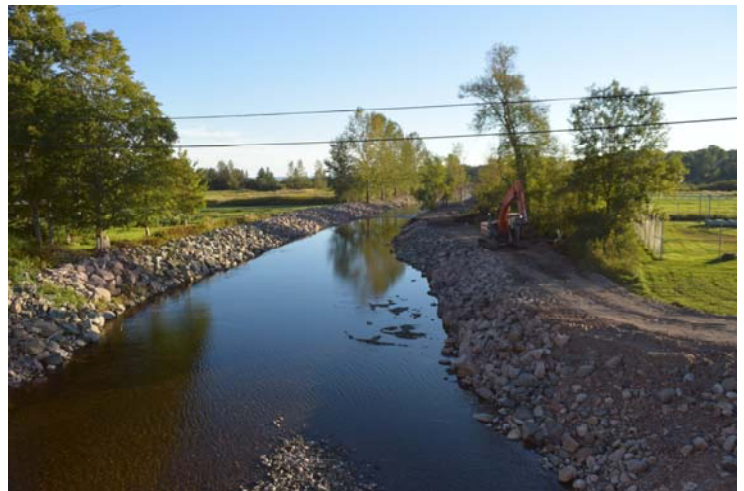
Great Village Channel Improvement
