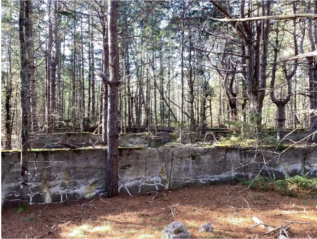
Image 7. Old foundations of Camp Debert (Stand 134, Debert Industrial Lands, Map 4).
