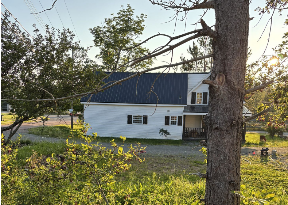
1792 Truro Road – Property to the west of subject property
