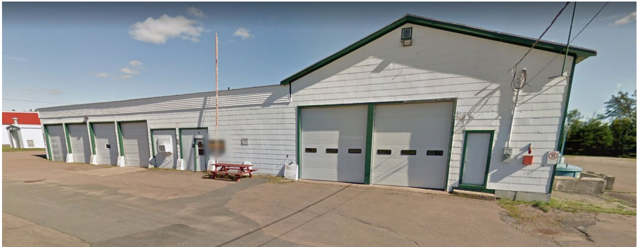
Street View – 15 Ventura Drive
